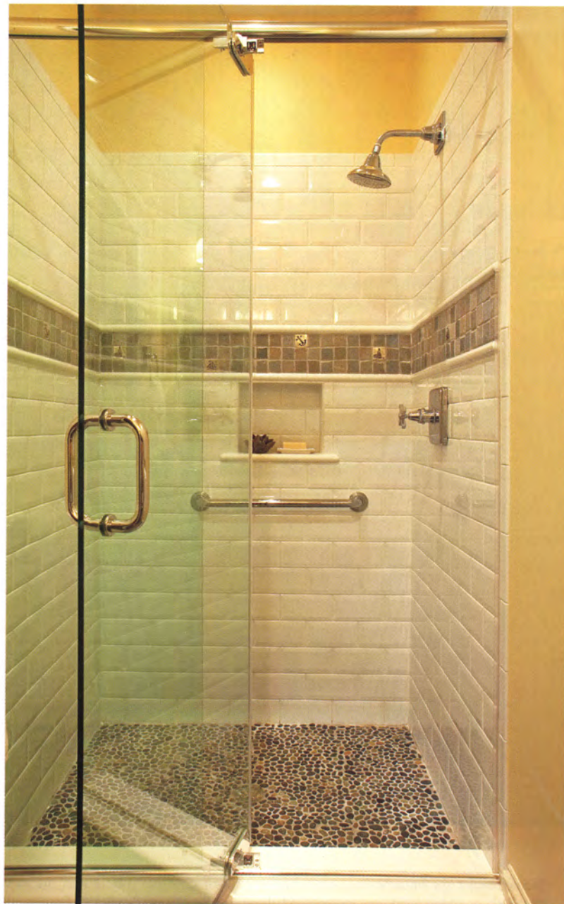
A river stone shower basin is complemented by white subway tile, and pewter inset tiles depicting shells and lighthouses.
